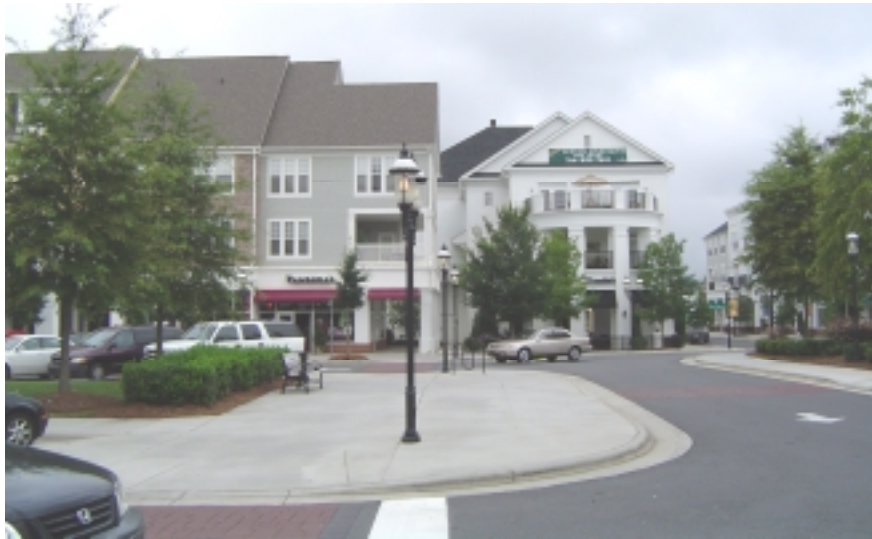
Birkdale Village, Charlotte, NC represents the type of new mixed use lifestyle center that could be developed near Northville's downtown.
