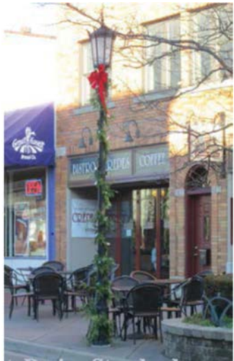
GFI receptacles located at the top of the pole
