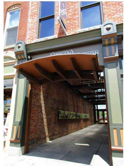
Photo: The Comerica Connection is another example of efforts to make Northville more pedestrian-friendly
