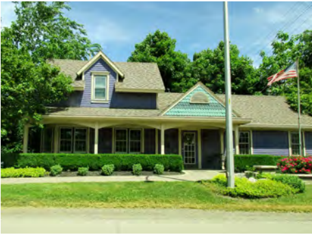
Photo: A high quality, well maintained structure near the Downtown core
