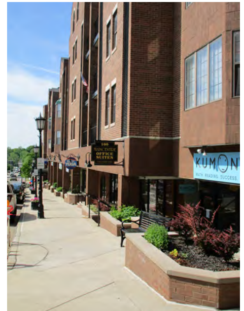
Photo: Streetscape in the central business district
