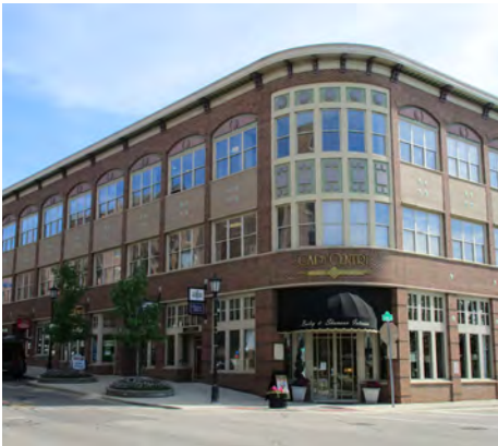
Photo: CadyCentre, a multi-story, brick building, is an example of Northville's great building stock and redevelopment potential
