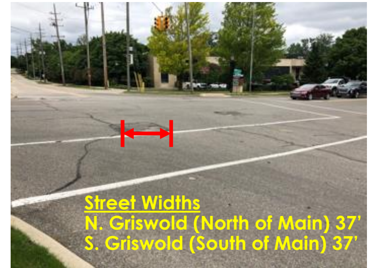
Figure 3E. Griswold and Main St. Crosswalks
