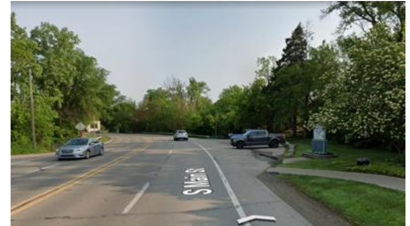
Figure 6D. S. Main entrance to downtown is a 4-lane curve (25 mph posted speed)
